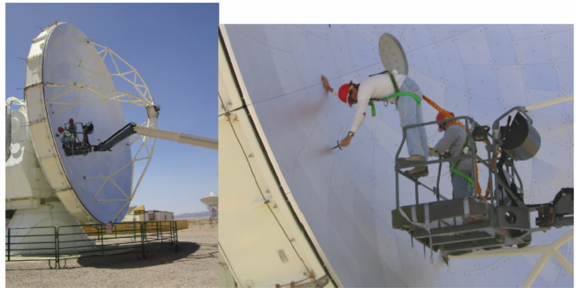
Fig. 9. Panel adjustment of the VertexRSI prototype antenna.
